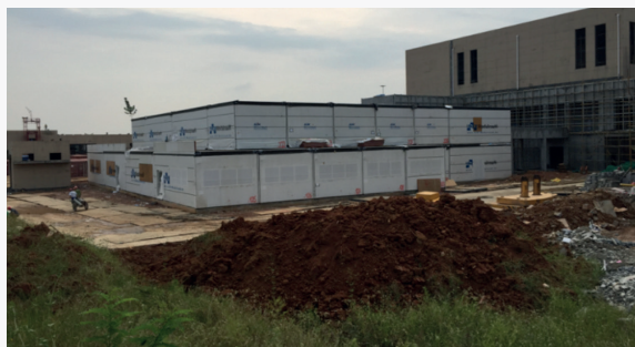
Figure 6: 62 modules in place after eight days
