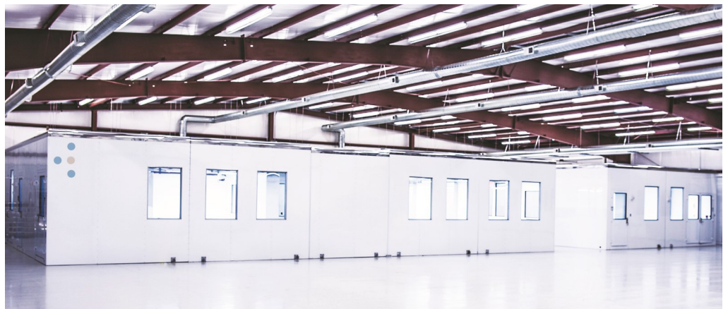
Figure 17: Traditional aseptic filling system within POD infrastructures
