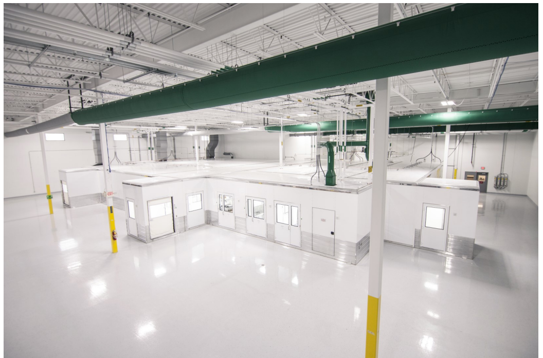
Figure 3: Cleanroom POD cluster (14 subPODs interconnected) for a gene therapy application
